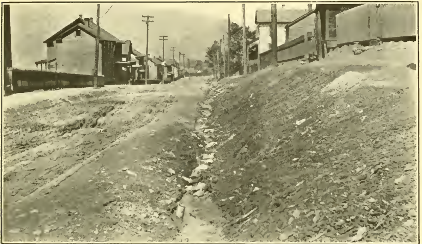
AN OPEN DITCH ALONG NEW STREET, PROSPECT.
